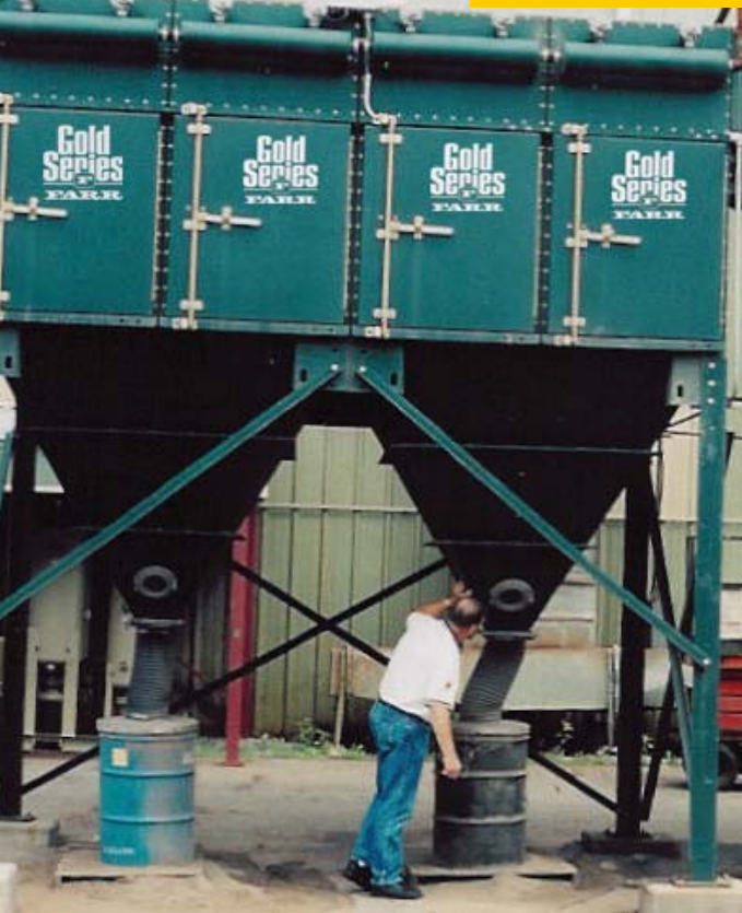
GS 48 on RR Car Sand Blasting
