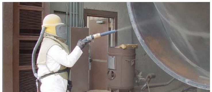
Room Air Blasting
